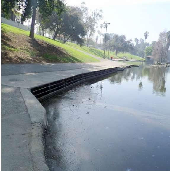
Figure 2-2. Northern Outlet/Inlet Structure Hollenbeck Park Lake Rehabilitation and Stormwater Management
