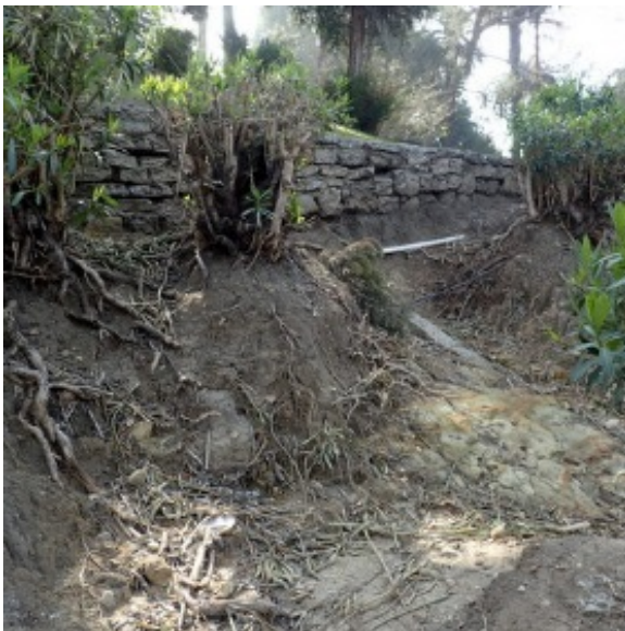
Figure 2-7-M. Hillside Erosion Exposing Irrigation Lines Hollenbeck Park Lake Rehabilitation and Stormwater Management
