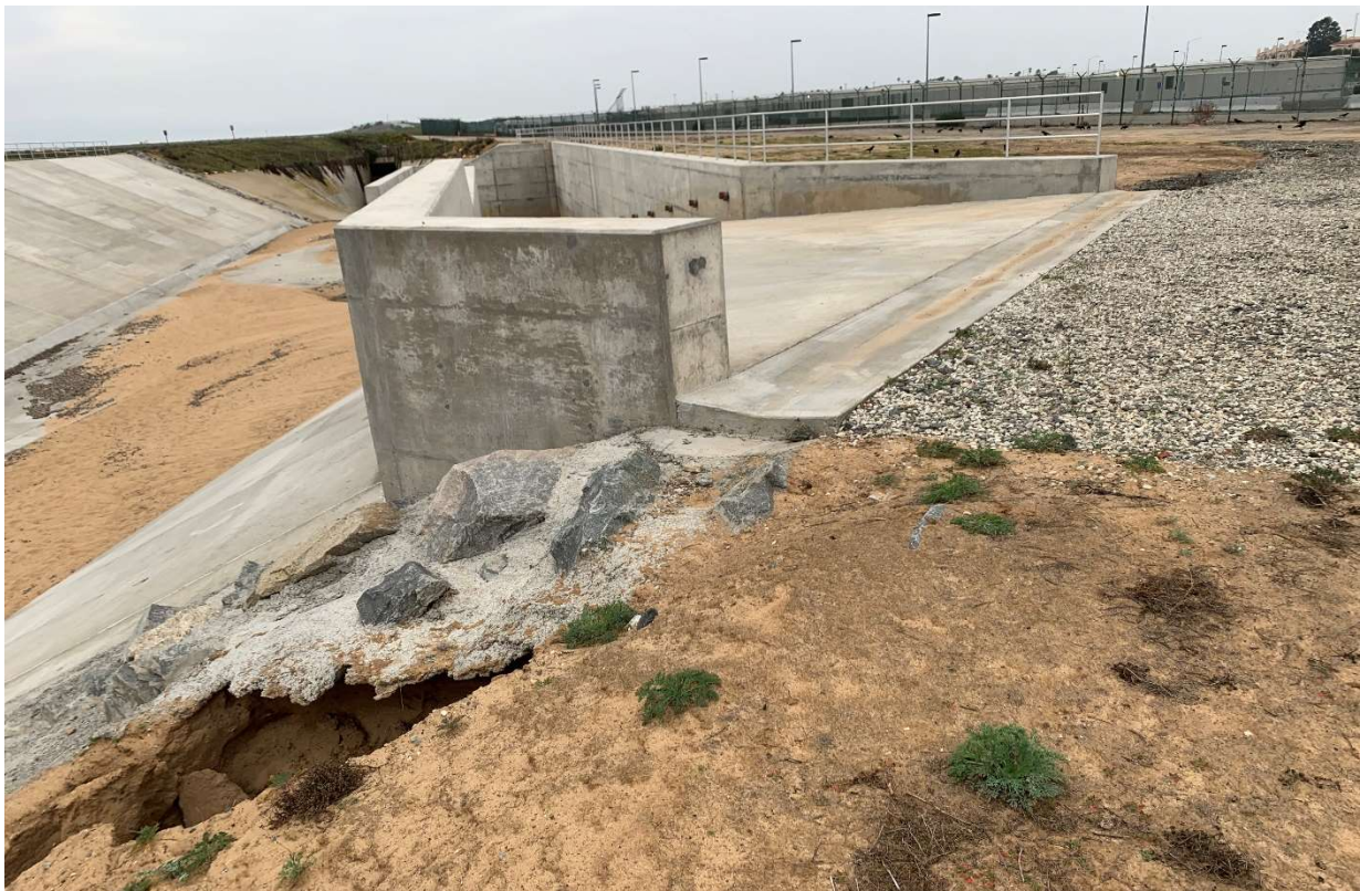
(Argo Drain Sub-Basin Facility)
