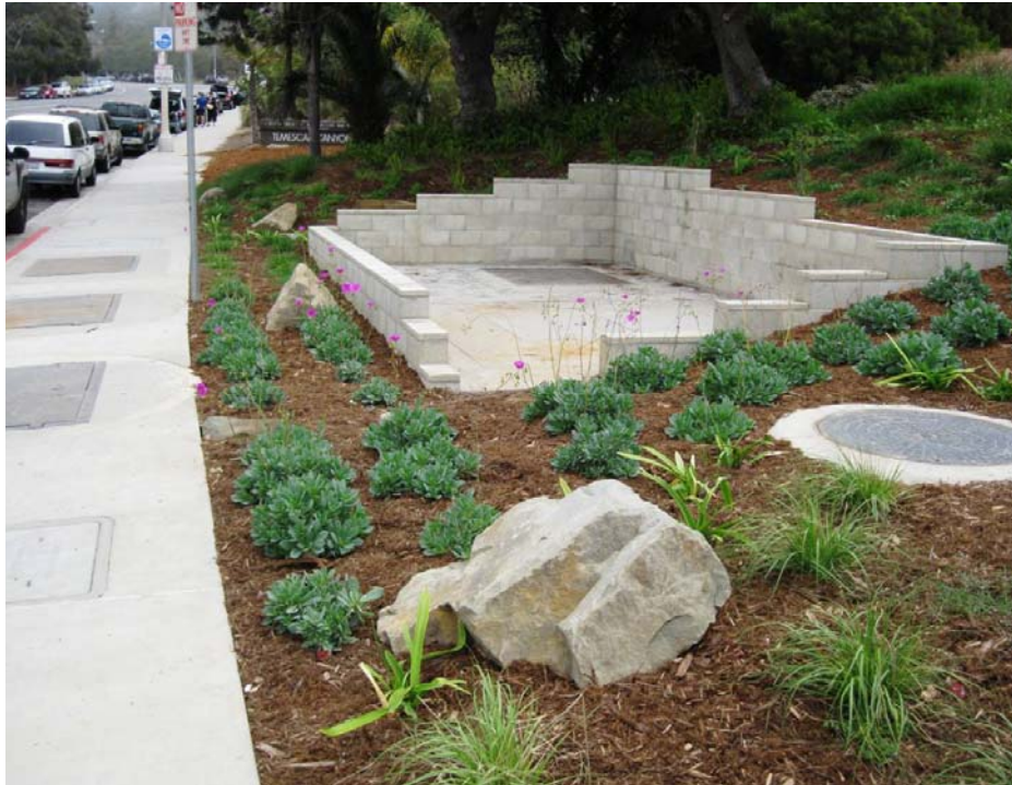
The completed Package 2 LFD Upgrade at Temescal Canyon Road
