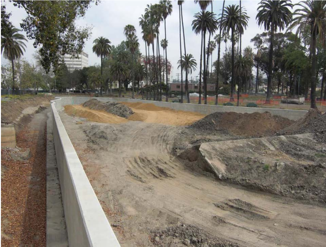
Retaining walls at Lotus Bed
