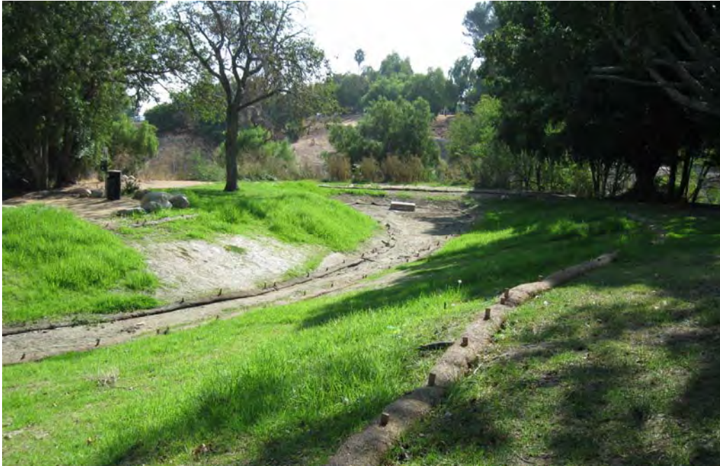
Bio-Retention basin at parking lot of Peck Park Canyon Project
